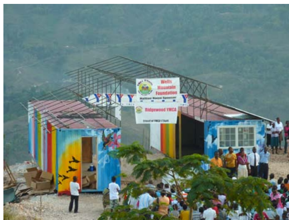
Still needing its roof, a few doors and some walls, the new YMCA of Laboule is dedicated at the end of our week in Haiti.
